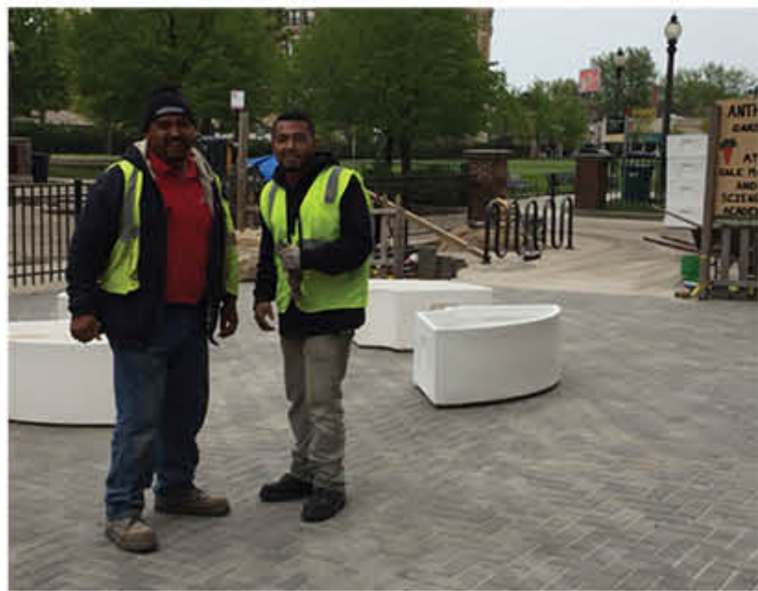
Christy Webber Employees Bring Big Green Beds in After Hardscaping
