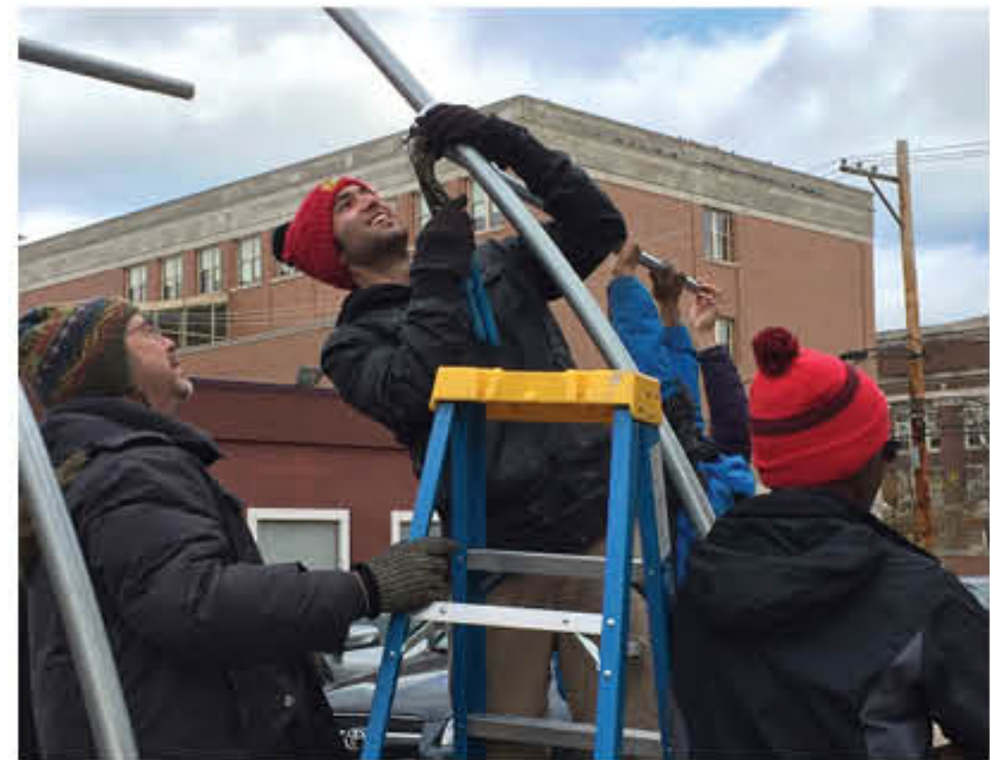
Volunteers Get Involved in Building the High Tunnel
