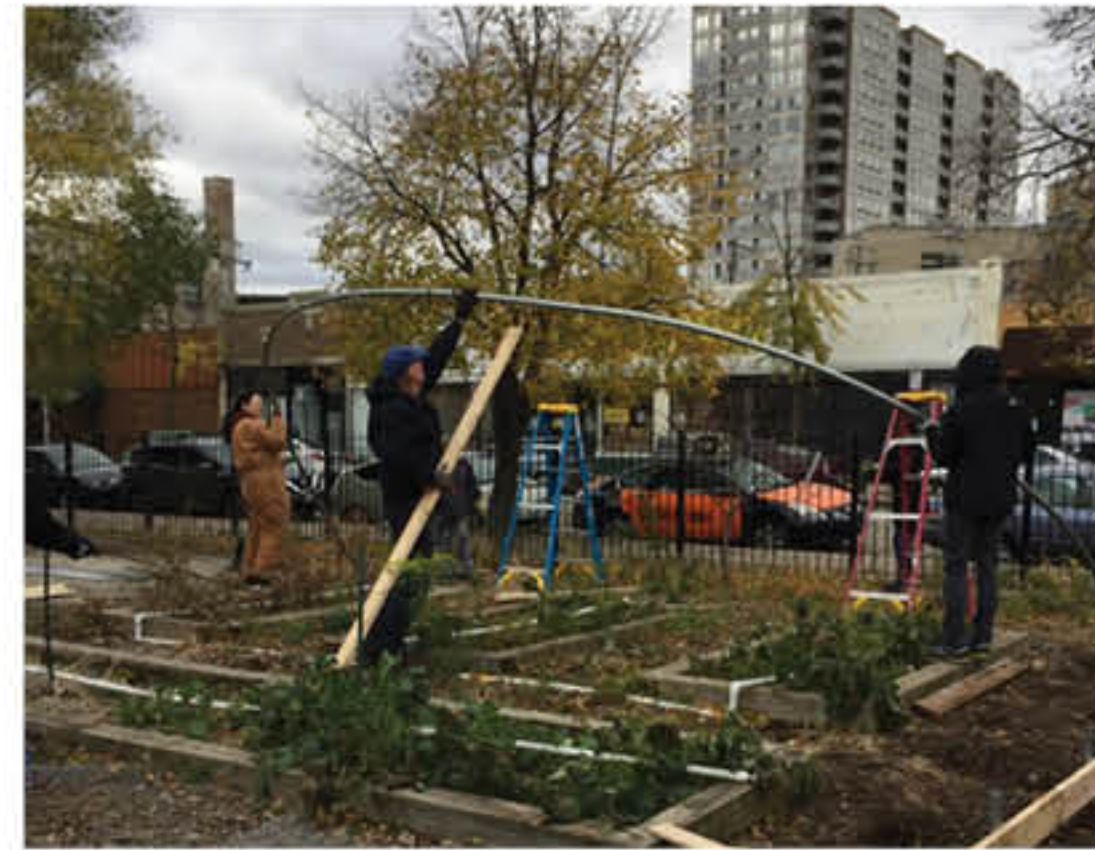
Progress is Made, Lifting the First High Tunnel Tubing Into Place
