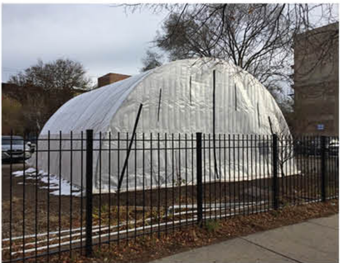
High Tunnel Construction is Completed, Ready to Grow Community Food
